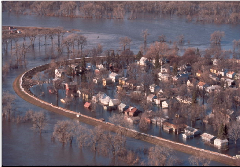
Areas behind levees which are overtopped or breached can experience significant damage and loss of life.
