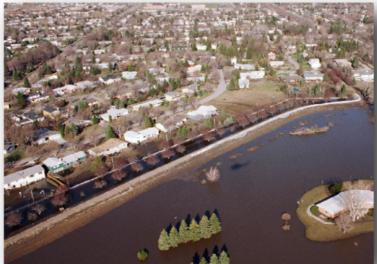
Accredited levees may help prevent properties from being flooded during the 1-percent-annual-chance flood.
